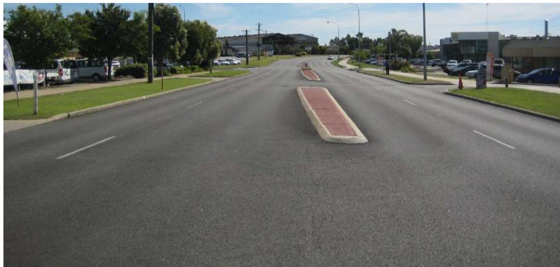
Figure 14: Collier Road looking west in the vicinity of the development site
