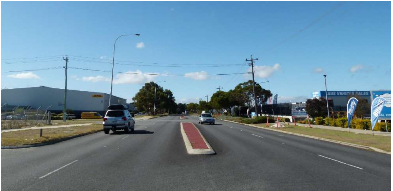
Photograph 3 – The dual-lane carriageway of Collier Road.
