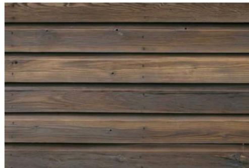
Horizontal weatherboard cladding
