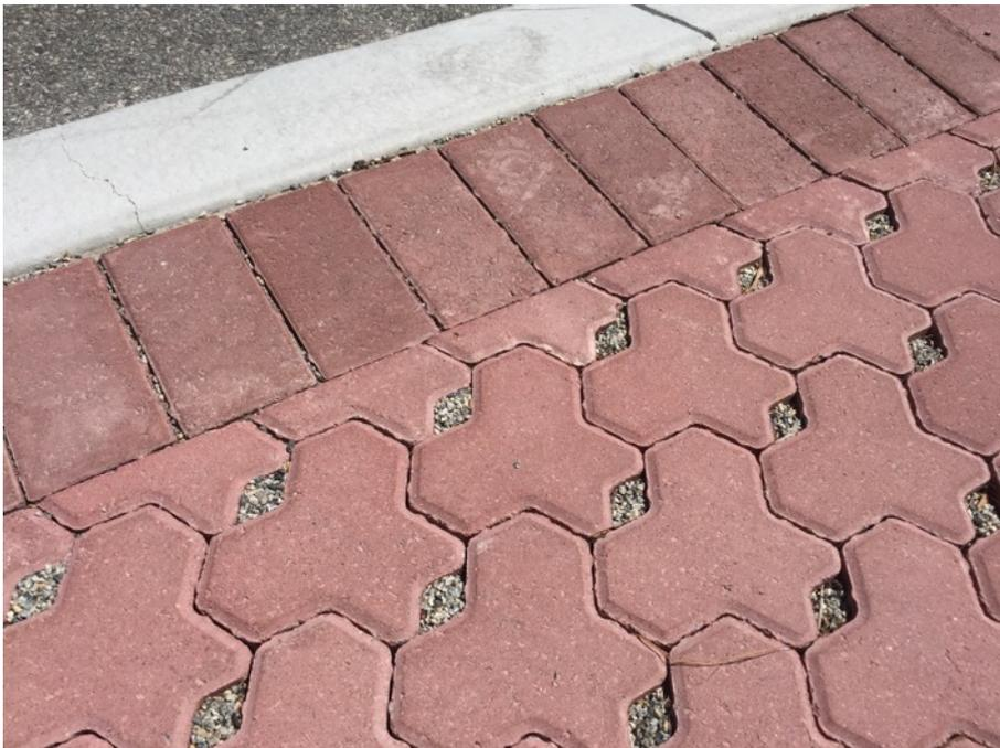
**Figure 8.** Permeable paving provides an option for hard surfacing that improves water infiltration and aeration to the soil profile (and tree roots) below, subsequently increasing tree growth rates and boosting performance.
