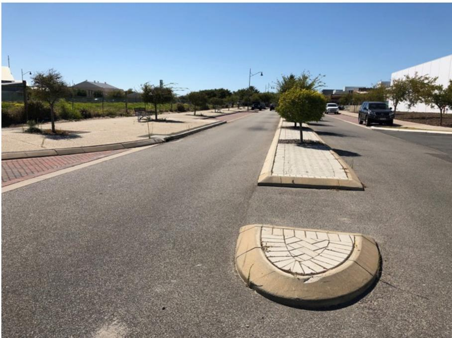
**Figure 12.** Placement of trees several metres away from the ends of the central median islands provides another technique to mitigate the potential for tree damage/ loss resulting from vehicle impact, and in doing so may reduce the total number of trees identified in the original design.
