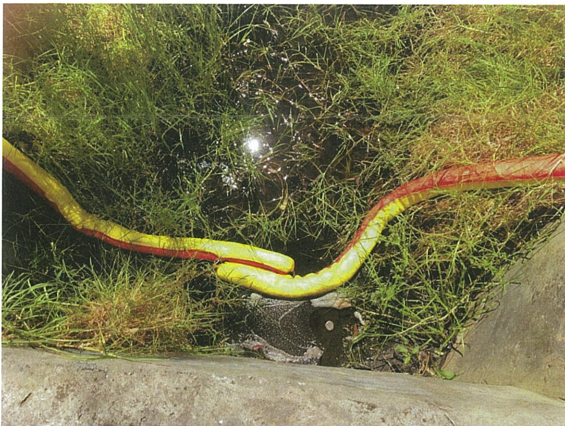
Photo 9 – Booms installed at the Swan River drainage outlet.
