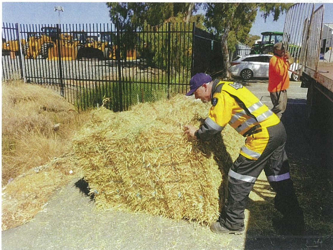
Photo 10 – DWER officer installing hay bales in the open drainage.
