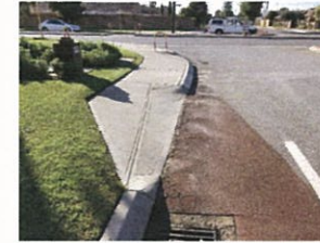
EXAMPLE OF CONCRETE CYCLING RAMP N.T.S.
