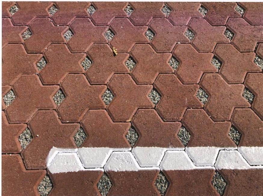
**Figures 7 & 8. Example of a pervious paving option to improve soil conditions and subsequent tree health.**
