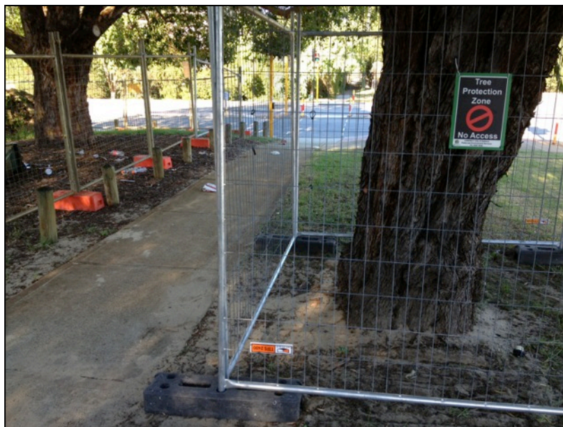
Figure 4. Example of protective fencing comprised of 1.8m high chain-wire mesh panels which should be erected at the TPZ periphery prior to the commencement of any construction activities that have the potential to collide with and damage the trunk and lower branches. Where site constraints restrict the erection of fencing at the TPZ periphery, the use of four panels (see above) should be considered the minimum tree protection requirement.
