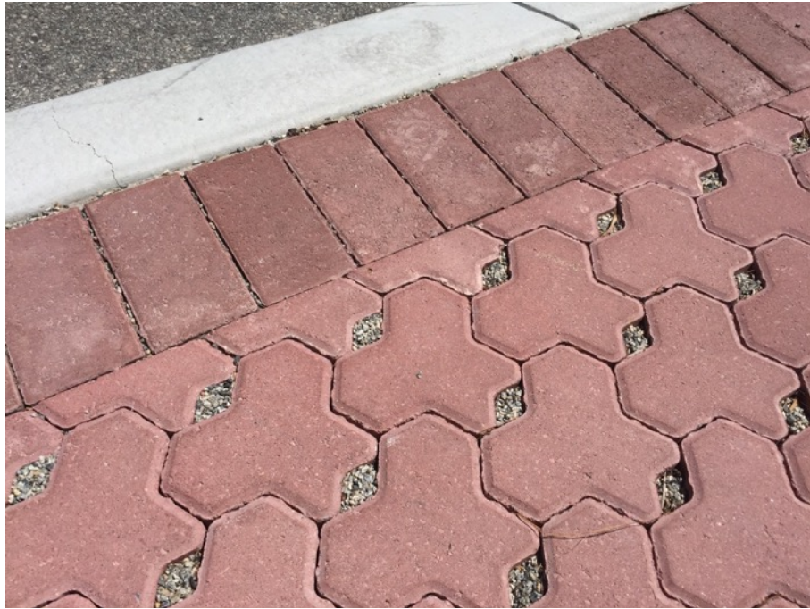
Figure 6. Where hard surfacing is proposed adjacent to existing trees the use of permeable paving provides an option to maintain and/ or improve water/ nutrient infiltration and adequate soil aeration (oxygen) to the small absorbing roots.
