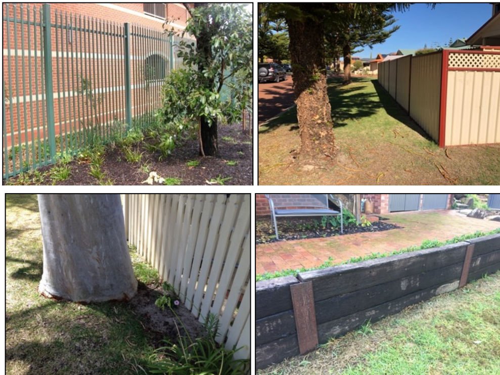
Figure 7. Example of root-sensitive options to span a wall or fence structure across the root plate of a tree whilst limiting excavation to avoid severing large woody roots: (a) Post and palisade fencing; (b) Post and panel colourbond fence; (c) timber picket fence; (d) i-beam and sleeper low wall.
