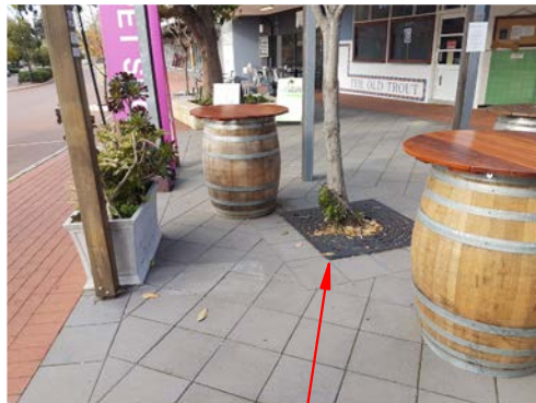
Remove Tree & Grate Make good / install paving
