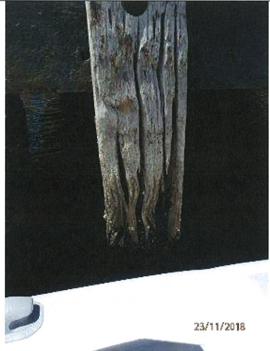
Photo 42 – View of the extensive weathering/cracks at the bottom of chafers.
