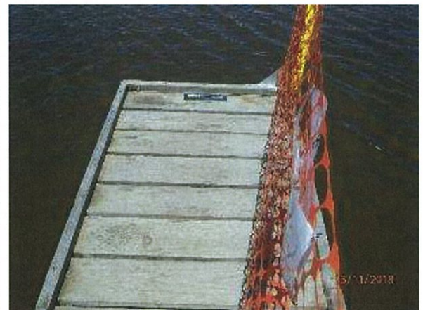
Photo 4 - Typical view of timber deck and kerbing.
