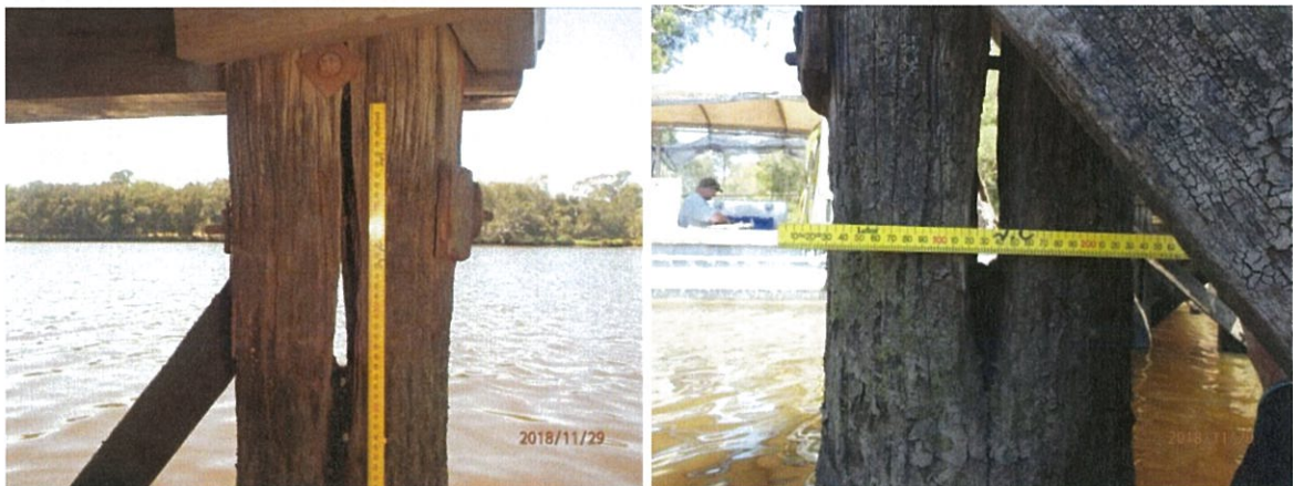
Figure 5: Shows vertical crack in outer western pile
