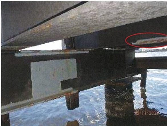
Photo 51 – Early spot corrosion evident to steel stringers on the bottom flange. Note: Previous paint repairs/patches were evident
