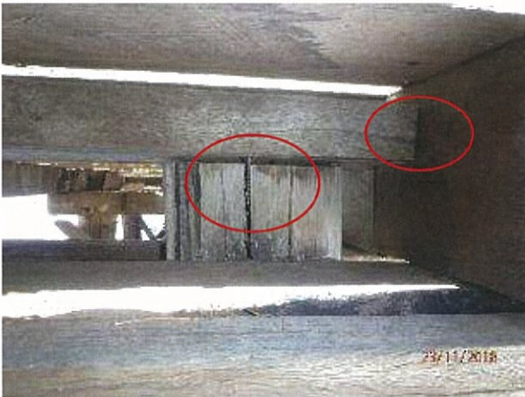
Photo 7 – Poor connection of timber stringer to pier, with split in timber at location of metal screws.
