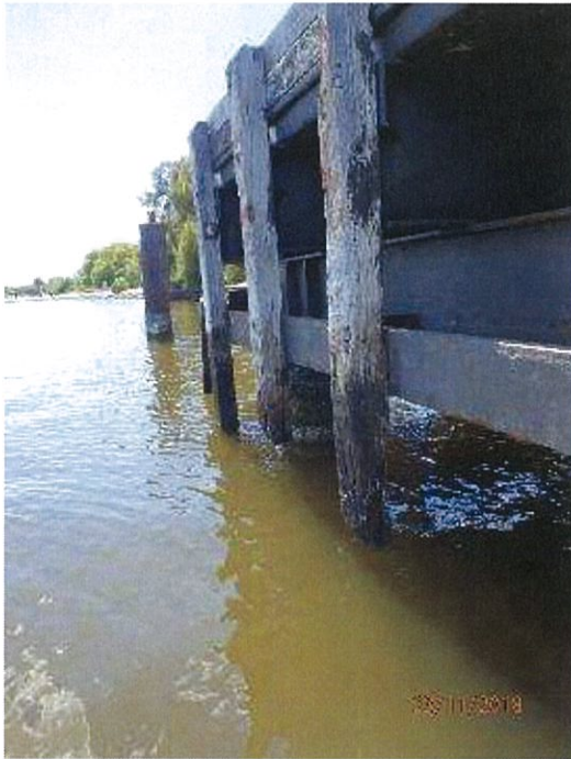
Photo 41 – Timber chafers along front of jetty have extensive weathering/cracks at the bottom.
