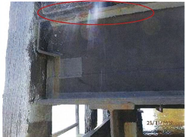
Photo 52 - Early spot corrosion evident to steel stringers on the top flange on external exposed faces. Note: Previous paint repairs/patches were evident.
