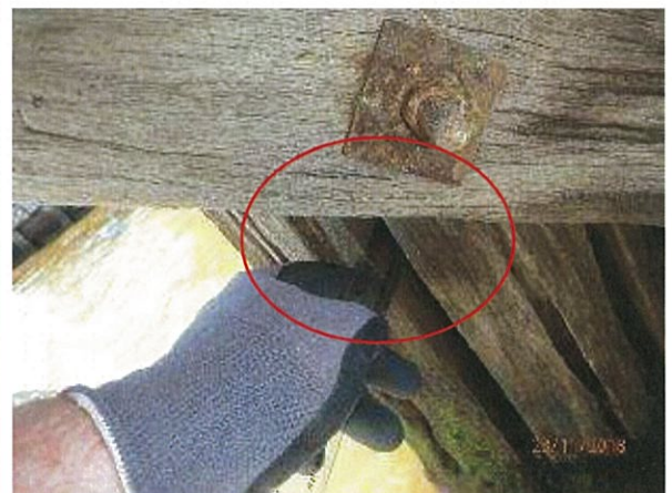
Photo 16 - Significant crack/section loss in timber pile on pier 2 with plastic ruler penetrating split across majority of pile diameter.
