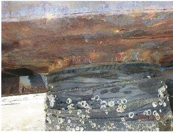
Photo 49 – Moderate corrosion evident to underside of the steel pile cap plates.
