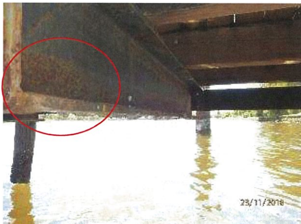
Photo 55 – Early spot corrosion was evident to the steel members supporting the timber decking on the low-level landing.
