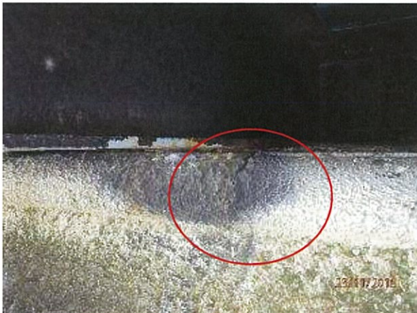
Photo 59 – A small crack was observed in the concrete seawall directly under the bearing area for the steel stringers.
