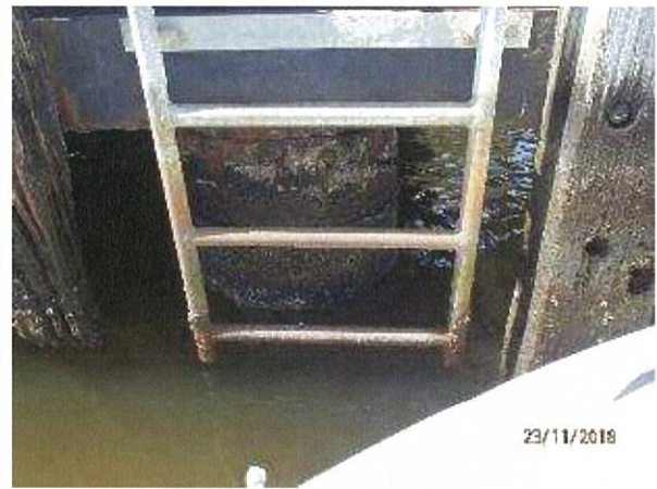
Photo 46 – Deterioration of galvanised coating and early corrosion on the bottom of ladder (in the tidal zone).
