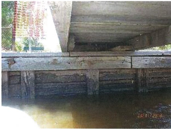
Photo 21 – View of underside of jetty deck at the shore connection, with extensive weathering, section loss and rot evident to shore timber retaining wall.
