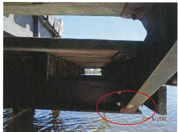
Photo 54 – Early spot corrosion was evident to the steel members supporting the stairs to the low-level landing.
