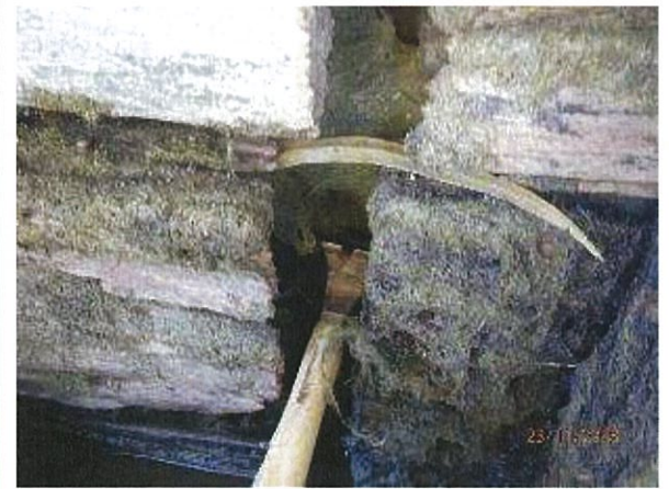
Photo 24 - Significant gaps were noted between longitudinal timber wall elements, exposing the filter cloth and potential loss of fill material from the shore.
