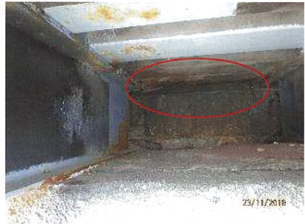
Photo 58 – Advanced corrosion was evident to the thin steel plate attached to the last steel sheet pile supporting the concrete deck (shore side).
