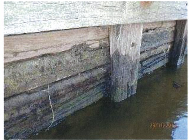
Photo 22 - Extensive weathering, splitting, section loss and rot evident to shore timber retaining wall on upstream side of jetty.
