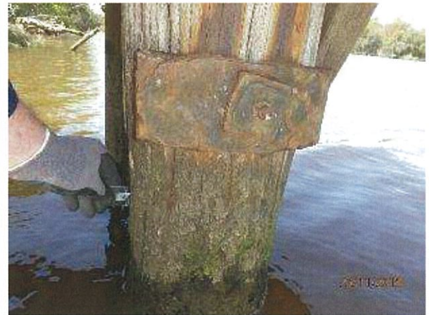
Photo 18 - Significant crack/section loss in timber pile on pier 3 with plastic ruler penetrating split across entire pile diameter.
