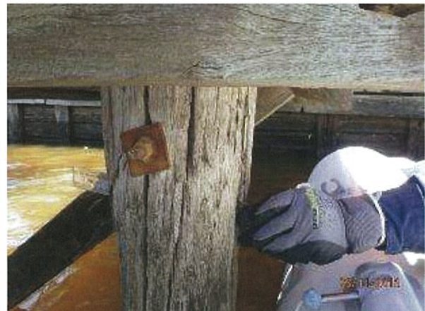
Photo 12 - Significant crack/section loss in timber pile on pier 1 with plastic ruler penetrating split across the entire pile diameter.
