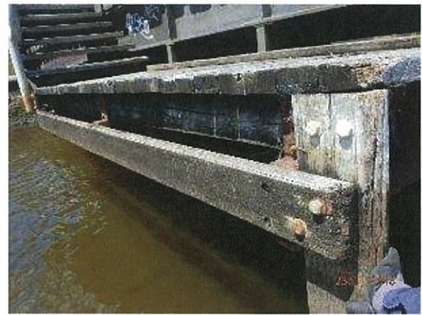
Photo 38 – The timber stringers (supporting timber deck boards), vertical timber chafers, and the timber waler beam on the low-level platform, all have evidence of significant weathering/splitting.
