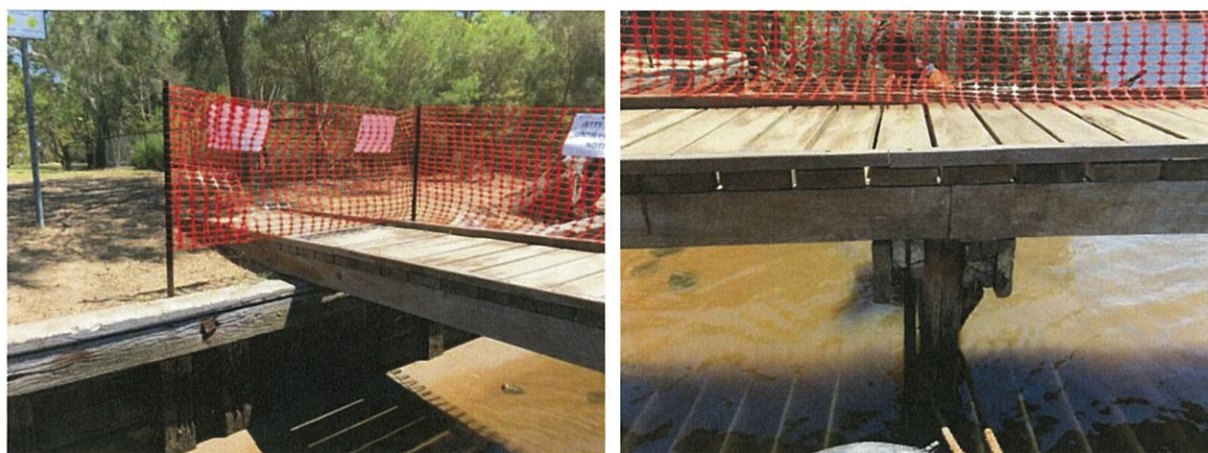
Figure 7: The two shoreside piles are smaller in diameter than the other four piles.
