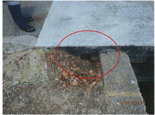
Photo 34 – Typical view of material loss at sides of jetty concrete slab connection with shore.
