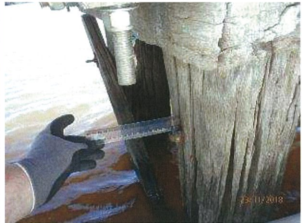
Photo 14 - Significant crack/section loss in timber pile on pier 2 with plastic ruler penetrating split across majority of pile diameter.
