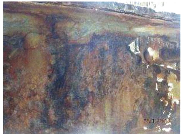
Photo 44 – View of steel water beam showing failed connection to timber chafer and significant corrosion/section loss.
