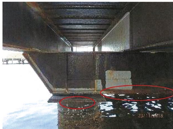
Photo 47 – Surface corrosion evident to top of steel pile cap plates and steel headstock beams.
