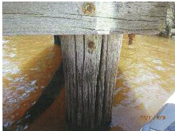
Photo 19 – Extensive weathering/section loss evident to external surface of timber pile on pier 3.
