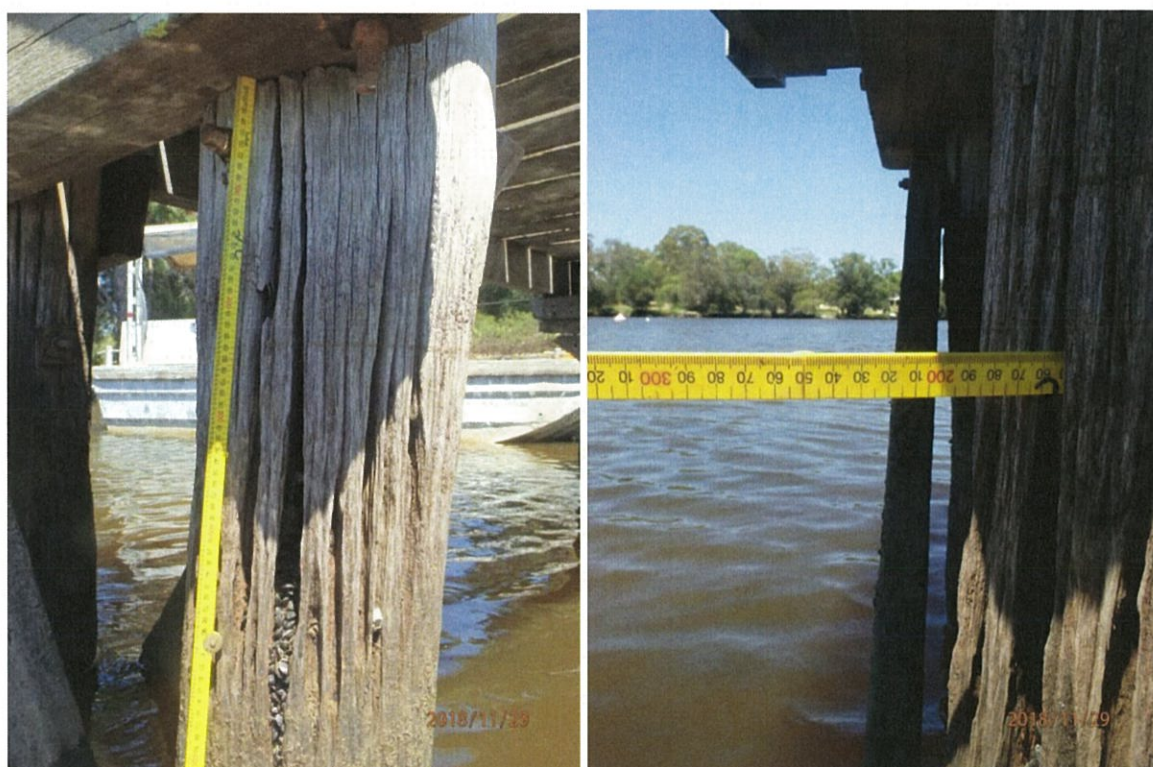
Figure 8: The extent of the cracking and splitting in the piles is obvious
