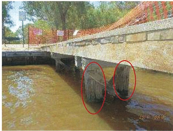
Photo 13 – View of central pier, with extensive weathering/section loss and large cracks/splits to external surface of timber piles.
