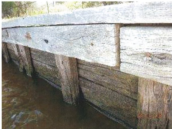
Photo 23 – Extensive weathering, splitting, section loss and rot evident to shore timber retaining wall on downstream side of jetty.
