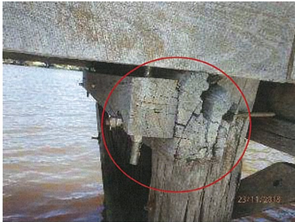
Photo 9 – Significant rot/section loss to original timber headstock beam and previous strengthening repairs to existing timber headstock, with additional timber beam bolted to side.
