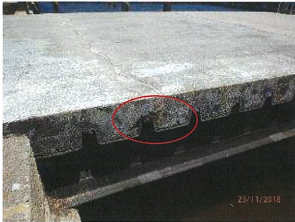
Photo 29 – Crack in concrete slab appears to be full depth to the supporting sheet pile steel sections located on the underside of the concrete deck.
