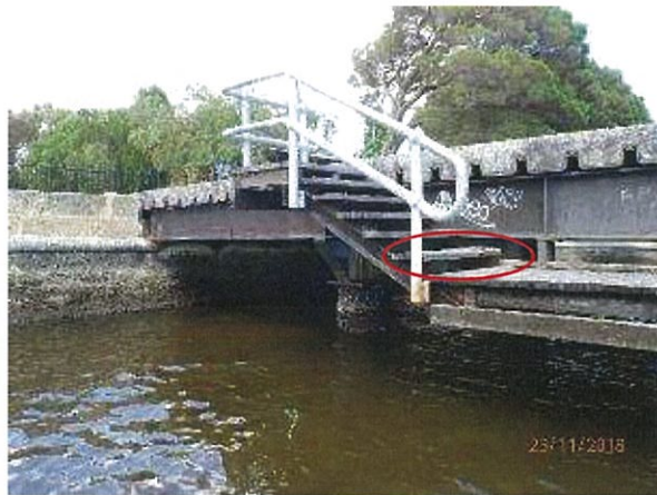
Photo 37 – Crack noted to lower timber stair tread.
