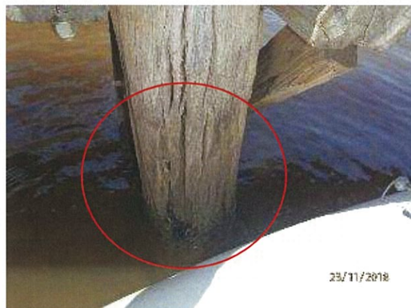
Photo 15 – Extensive weathering and section loss evident to external surface of timber pile on pier 2.
