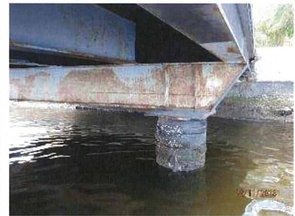
Photo 48 – Surface corrosion evident to steel pile cap plates, steel headstock beams, and steel stringer beams.
