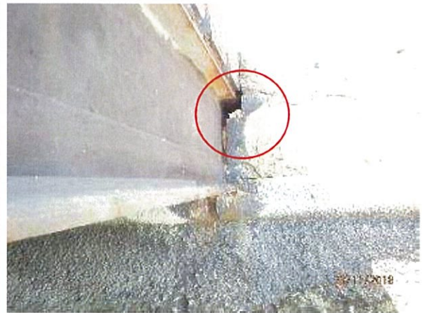
Photo 60 – A small hole was observed at the shore connection of the outside steel stringers and the limestone retaining wall.
