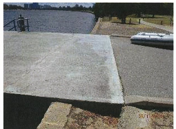
Photo 28 – Shore connection with jetty concrete slab. Note: Crack evident in slab top surface due to differential settlement in supporting structures.
