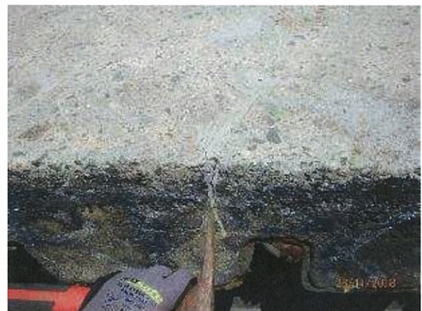
Photo 32 - Previous "V type" repairs to fine cracks in the concrete deck slab. Fine cracks in concrete slab appears to be full depth to the supporting sheet pile steel sections.
