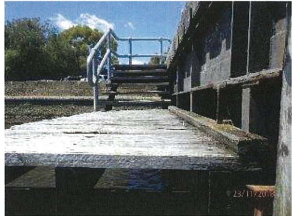
Photo 36 - Timber deck boards on the low-level platform appear very dry and require oiling/sealing.
