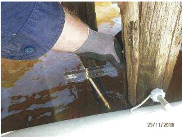
Photo 11 - Significant crack/section loss in timber pile on pier 1 with plastic ruler penetrating split across majority of pile diameter.
