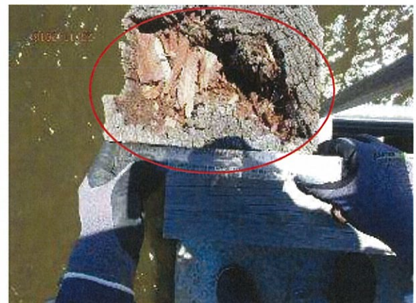
Photo 40 – Timber chafers unsealed at the ends with advanced rot/section loss in the top.
