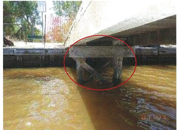
Photo 10 - View of near shore pier, with significant section loss/weathering on external surface of timber piles resulting in limited effective pile diameter supporting the jetty.
