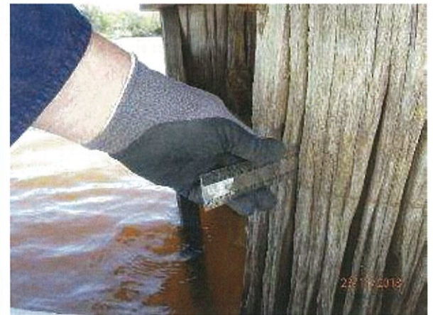
Photo 20 - Significant crack/section loss in timber pile on pier 3 with plastic ruler penetrating split across majority of pile diameter.
