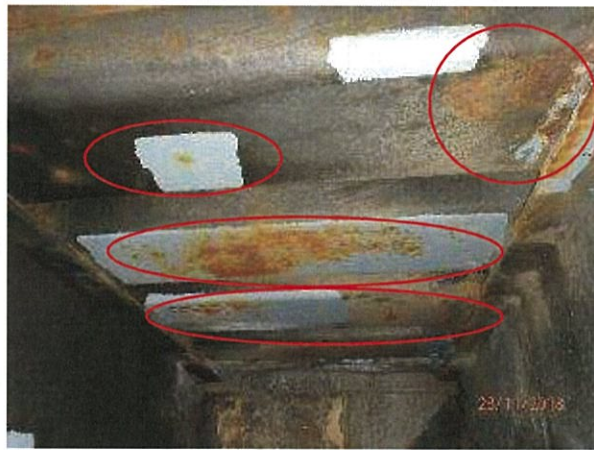
Photo 53 – Early spot corrosion was evident to the steel sheet pile members on the underside of the concrete deck. Note: Previous paint repairs/patches were evident.
