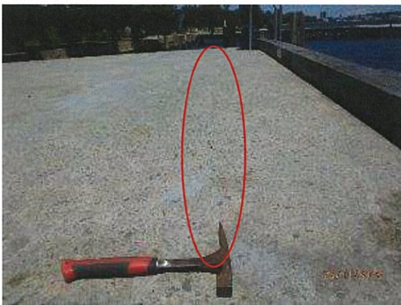
Photo 31 - Previous "V type" repairs to fine cracks in the concrete deck slab.
