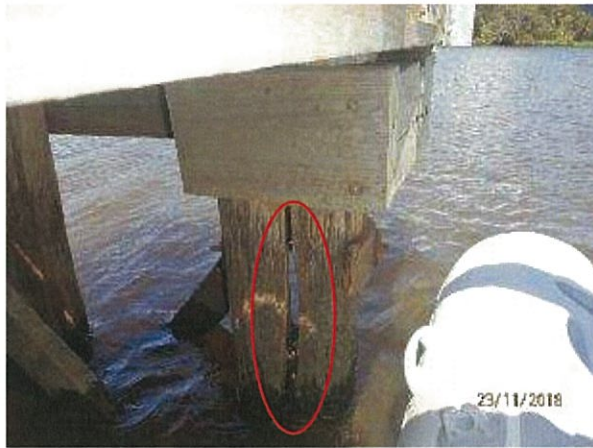
Photo 17 – View of end pier, with large crack with extensive weathering/section loss to internal section of pile.
