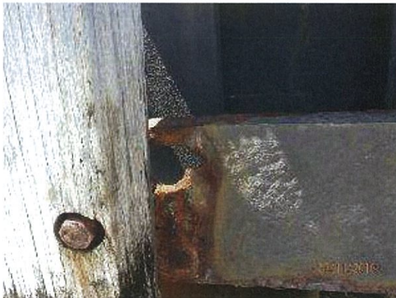
Photo 43 – Hole in steel water beam on the front of the jetty supporting the timber chafers.
