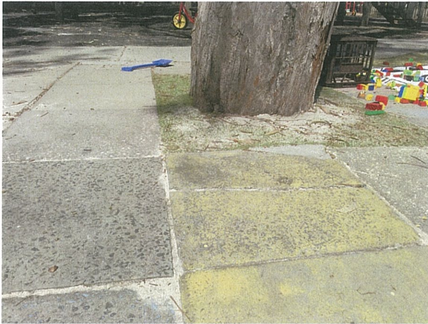
Figure 7. Concrete slab pavers were visible as the surface treatment with closer inspection revealing cracked pavers as well as displacement by approximately 10mm, typical where hard surfacing is located in close proximity to mature trees; looking towards the east.
