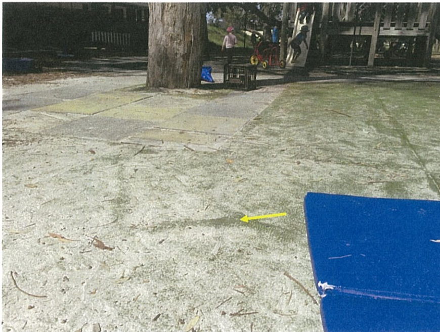
Figure 8. A root/ surfacing conflict was observed on the southwest side (see arrow) at a distance of 3.3m from the tree, with the root size estimated to be 20mm in diameter; looking towards the northeast.
