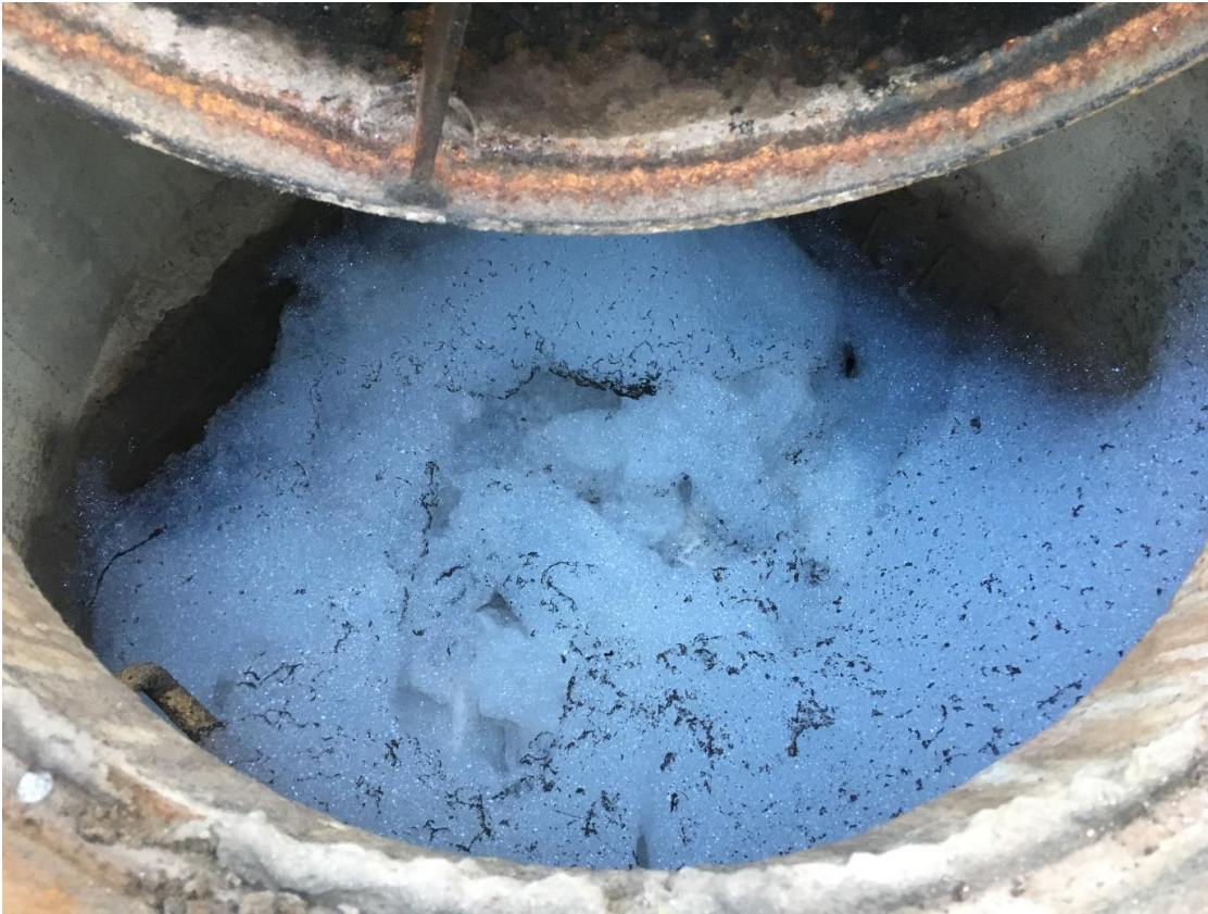
Photo 7 - Foam observed inside City of Swan stormwater system.
