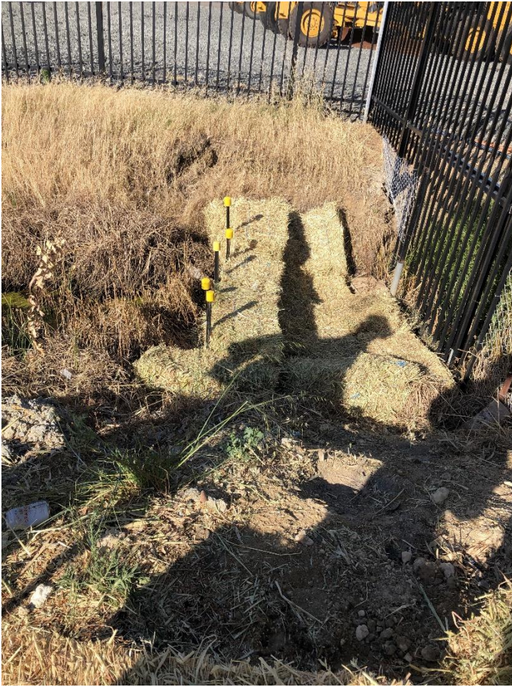
Photo 11 – Installed hay bales near to Great Eastern Highway, South Guildford.
