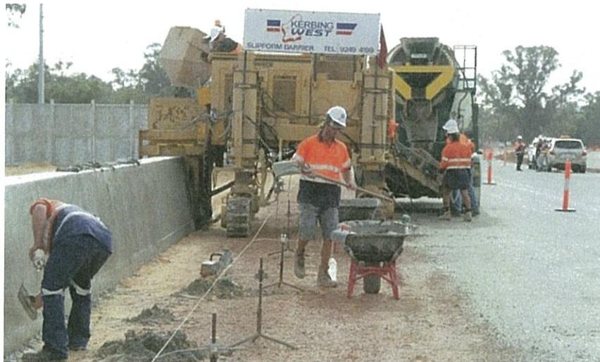
Figure 6: Typical machinery for slipform barrier construction
