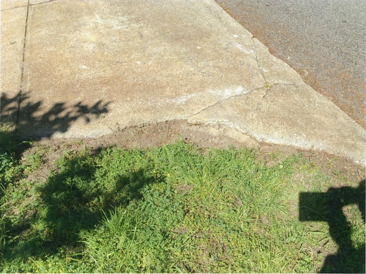
Photo of the crossover and the verge after being hit by the truck and after removing the retaining wall
