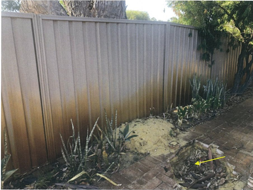
Figure 5. Displacement of the paving was evident within the property on the west side of the fence and previous lifting of the pavers revealed a large woody root of approximately 180mm diameter (see arrow) within the structural root zone of the tree; looking towards the southeast.
