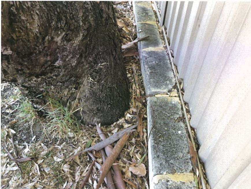
Figure 8. Near-contact between the root collar and fence was observed and subsequent minor displacement of the limestone low block wall foundation and upper colourbond post and panel fence was evident; looking towards the south.
