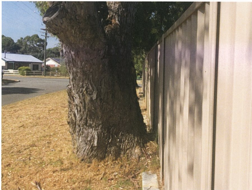
Figure 4. Contact between the root collar and fence was observed and subsequent displacement of limestone low block wall foundation and upper post and panel fence was observed; looking towards the south.
