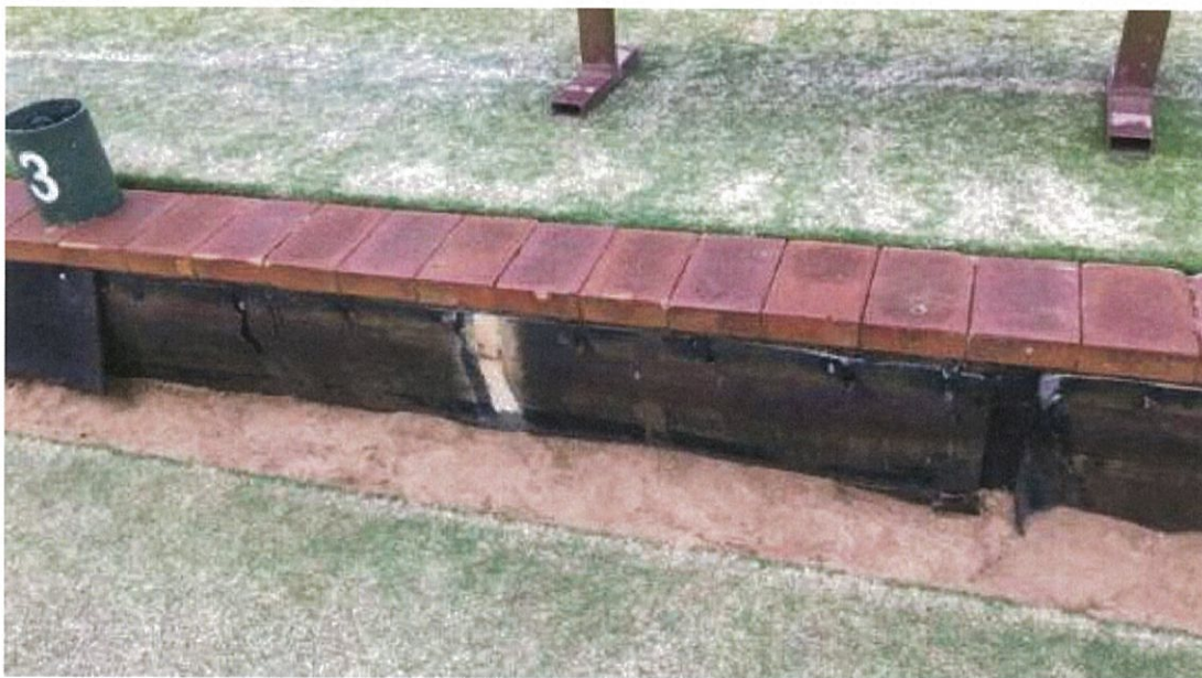
Damaged and degraded apron protection at corner tie in with earlier repaired section of apron
