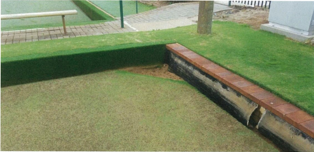
Damaged and degraded apron protection at corner tie in with earlier repaired section of apron
