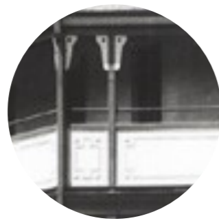
02 Re-instate timber post details
