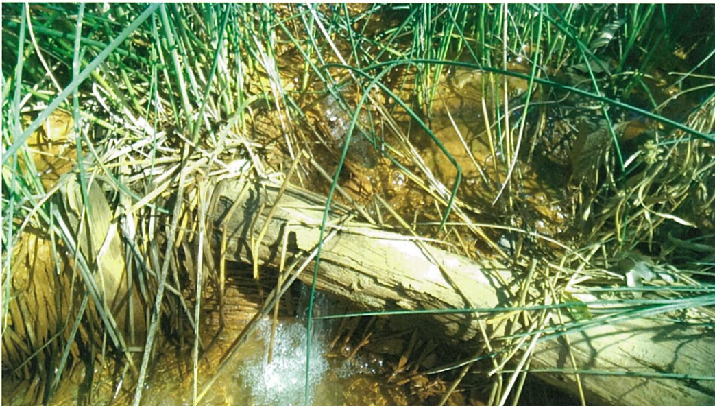
Photograph 4: Natural spring outflowing on the western river embankment upstream of the drainage outflow structure.
