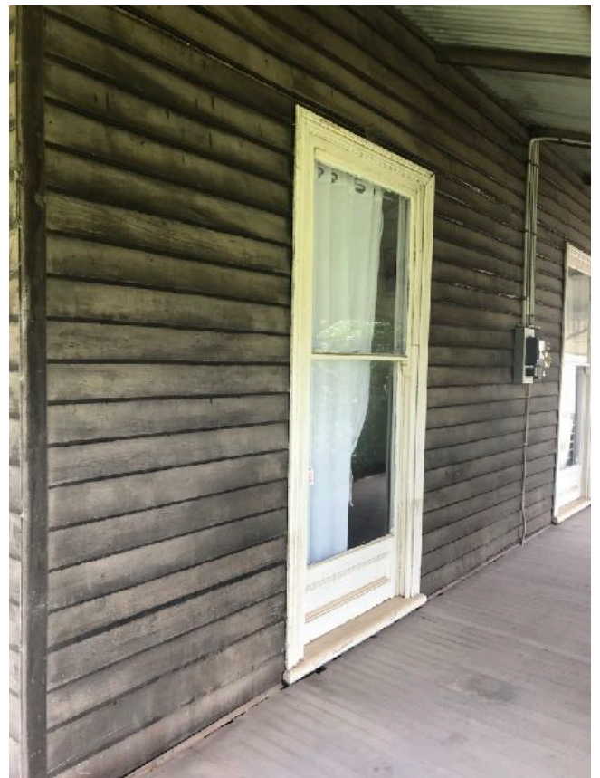
FRONT COLONIAL SASH WINDOWS
