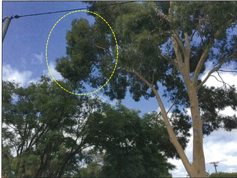
Figure 6. The previous branch failure from the lower crown on the southwest side has resulted in the residual foliage for the first order structural branch extending southwest over the residential property being concentrated at the distal section of the branch (see dashed line), subsequently reducing the ability of the branch to mass dampen/ dissipate wind loads; looking towards the southwest.
