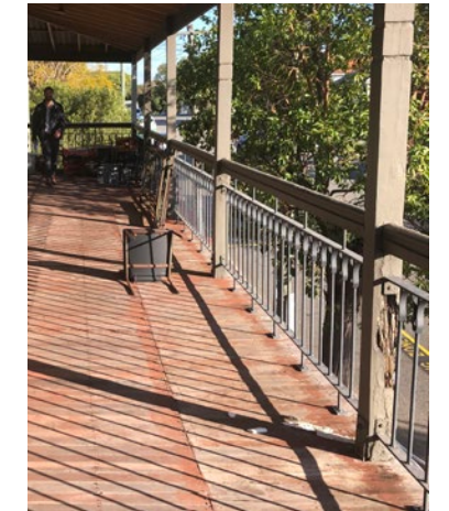
Existing balustrade to be retained, new clear panel applied at the back for compliance.
