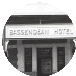
03 Re-instate signage in the style of the original c.1929/ 'Framed frieze' detail
