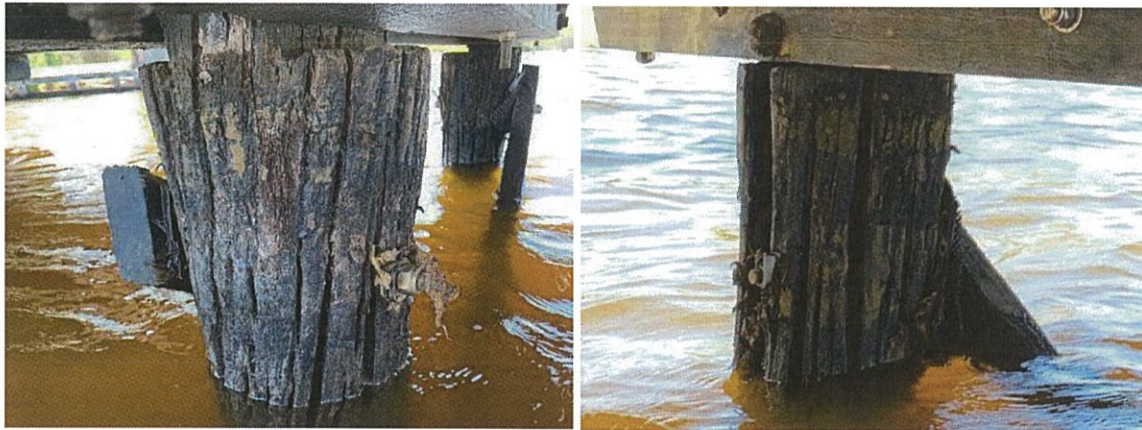
Figure 2.1 Piles – Above Water Portion
