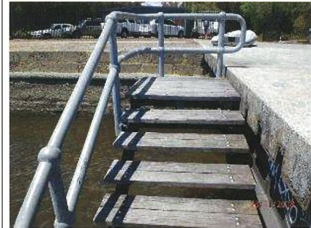
Photo 35 - Timber decking and galvanised handrail on stairway to low-level platform.
