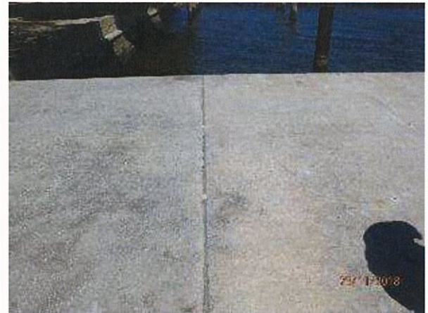
Photo 30 – View of existing construction joint in concrete deck slab.
