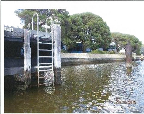
Photo 45 – Front ladder access to jetty.
