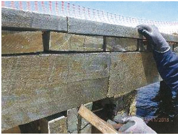
Photo 5 – Typical view of timber stringers supporting the timber deck planks.
