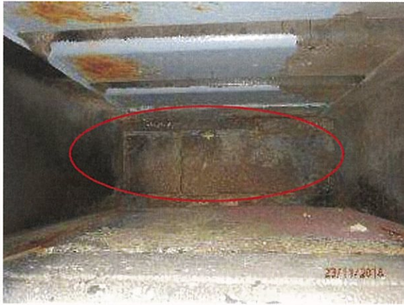
Photo 57 – Fretting of mortar was evident to the limestone retaining wall at the shore connection of the jetty.
