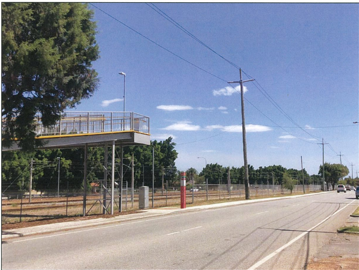
OVERHEAD POWERLINES ALONG RAILWAY PARADE
