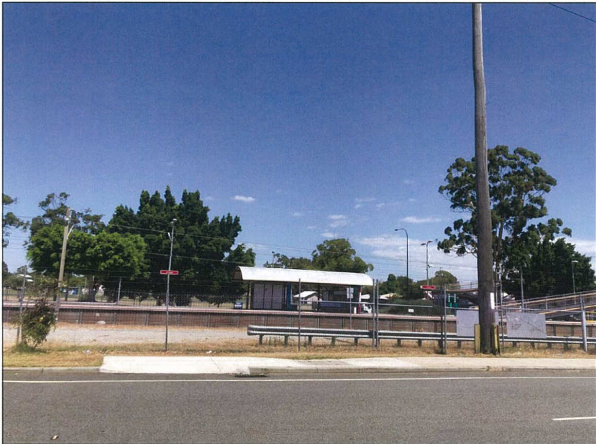
ASHFIELD STATION – VIEW FROM RAILWAY PARADE
