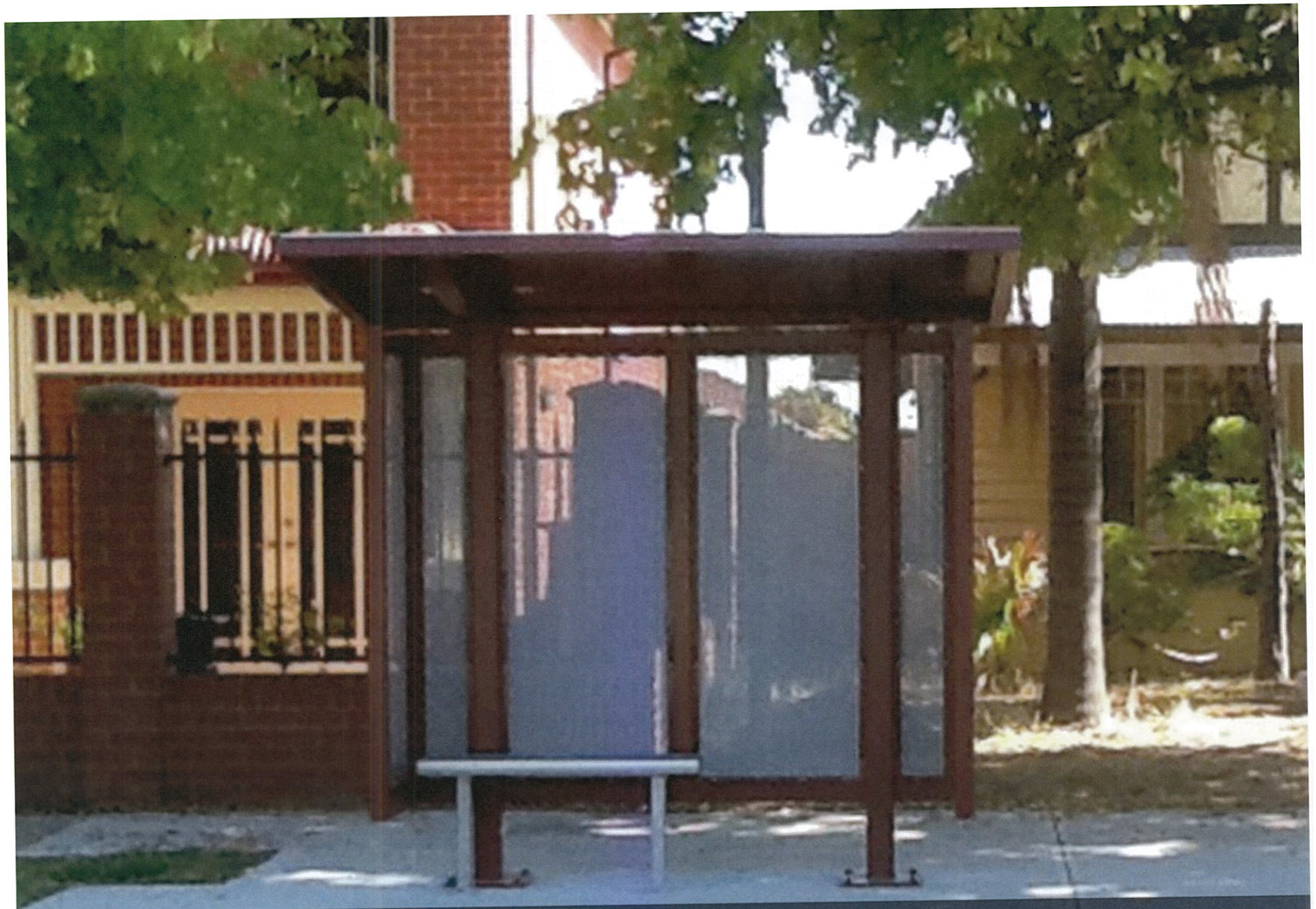
JSG MINI Bus shelter by Jason Signmakers. PTA Subsidy Approved
