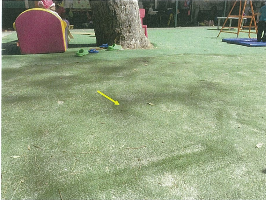
Figure 5. A root/ surface conflict with root of approximately 40mm in diameter was evident on the north side (see arrow) at a distance of 2.8m from the tree.
