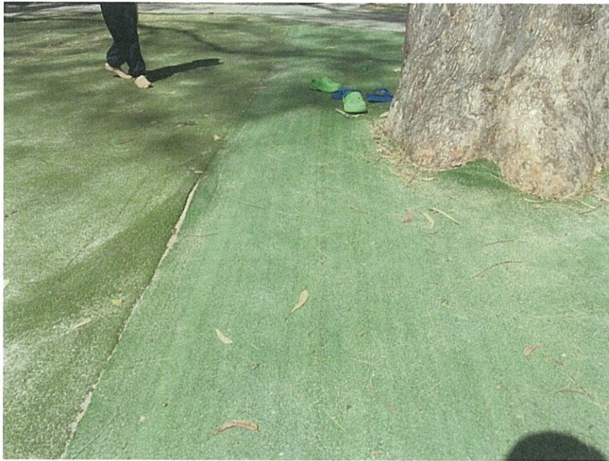
Figure 3. Fill soil of an estimated 200mm in depth is likely to have been applied atop the original soil level during the previous installation of the synthetic turf surfacing; looking towards the east.
