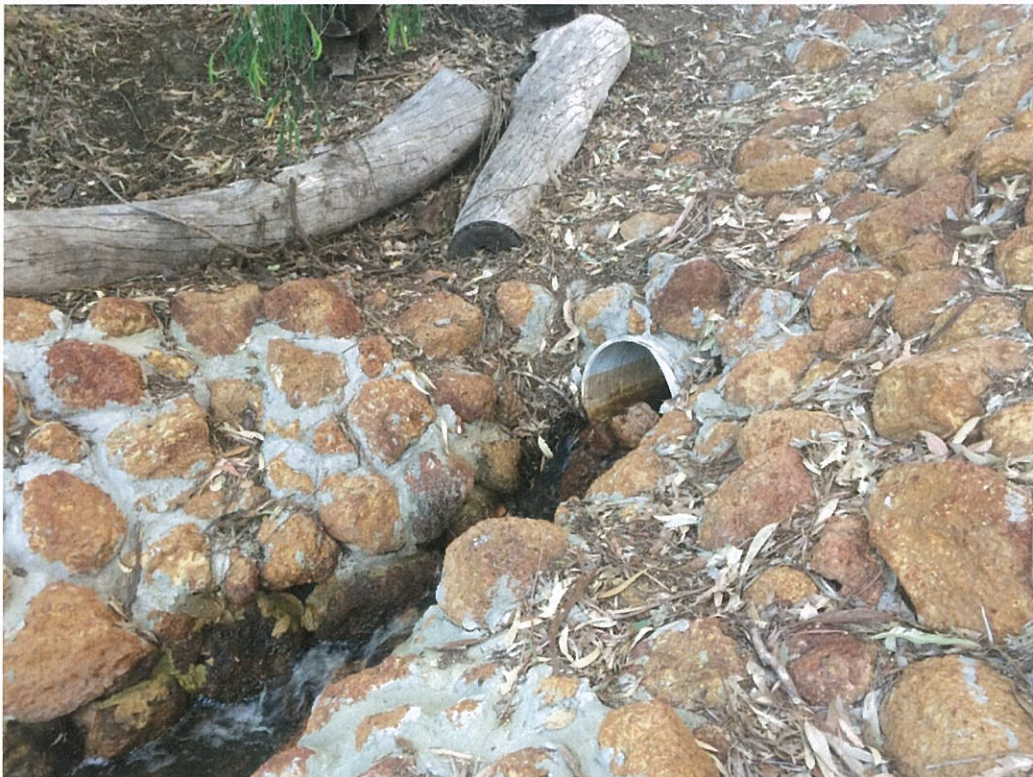
Photograph 2: Outflow pipe at the top of the embankment.
