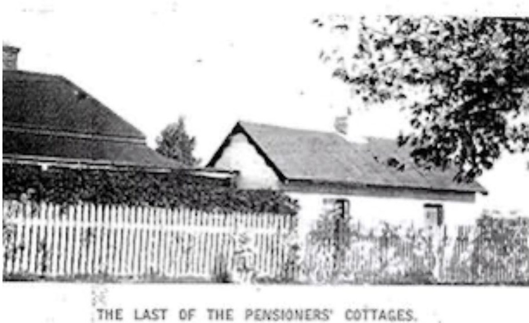
Figure 1. Pensioner Guard Cottage showing the c.1893 Residence on the left. Alf Thomas, History of Bassendean, 1947, p.13. Conservation Management Plan 2007.
