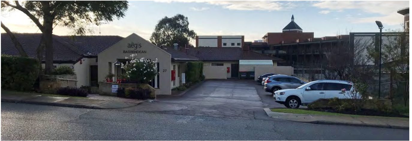
Photograph 1: Looking east from Hamilton Street at the existing Aegis facility on Lot 54.
