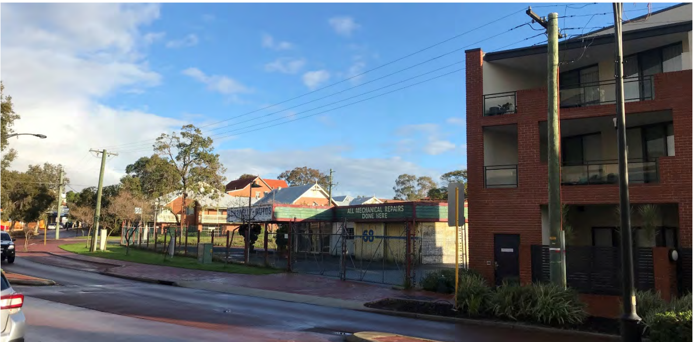
Photograph 5: Looking north west at the dilapidated buildings on Lot 85 Old Perth Road and more recent adjacent apartment development (Whitfiled).
