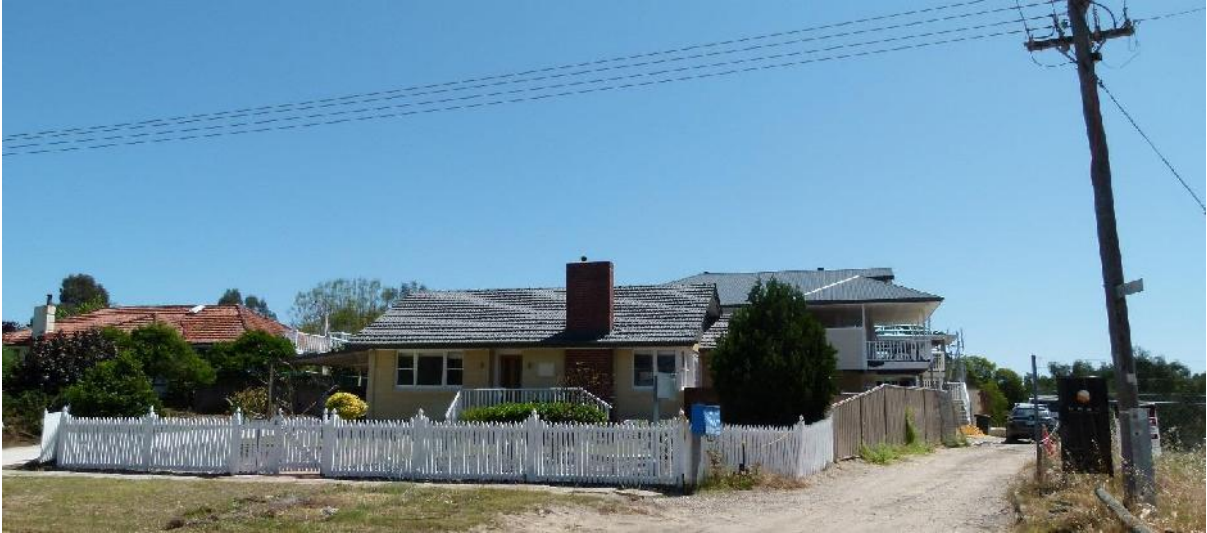
Photograph 7: Two storey development under construction, approximately 57m east of the subject site.
