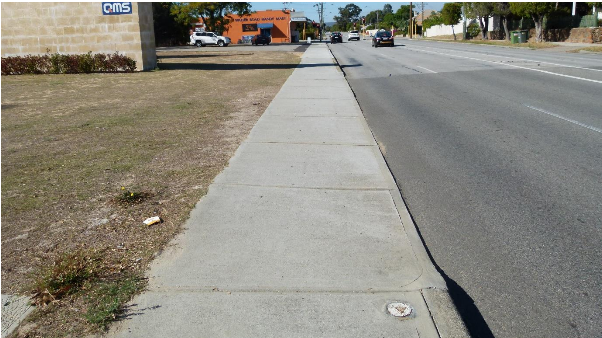
Photograph 5 – Existing pedestrian path and crossover to Walter Road East.
